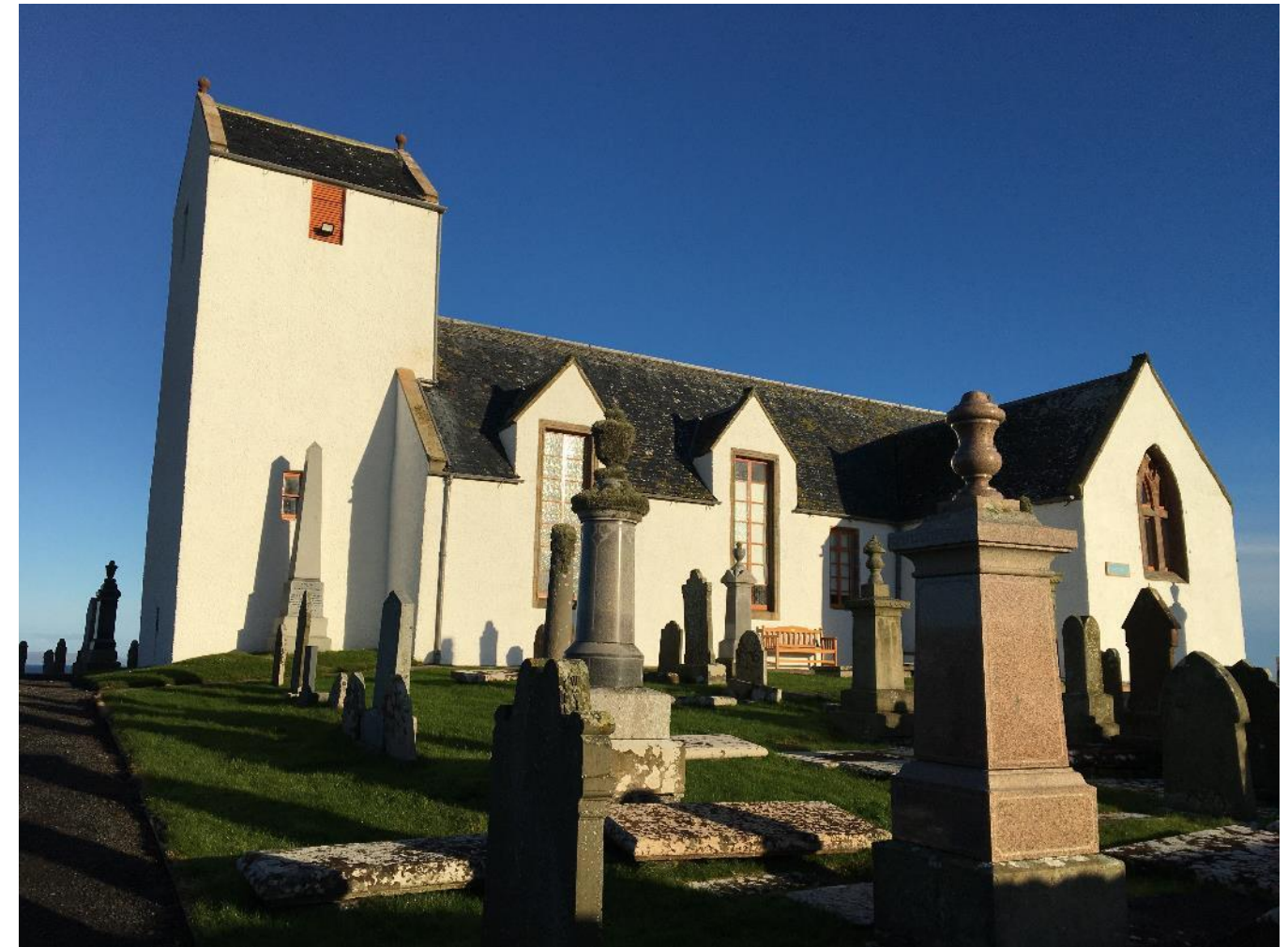
Figure 11.27. Canisbay Parish Church LB1795, looking north
